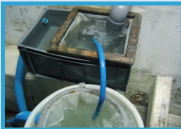
FIGURA 2.8. Colector de desagüe (Global Aquafish).
