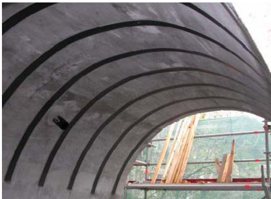
Figure 2.6. FRP strengthening of a masonry barrel vault.
