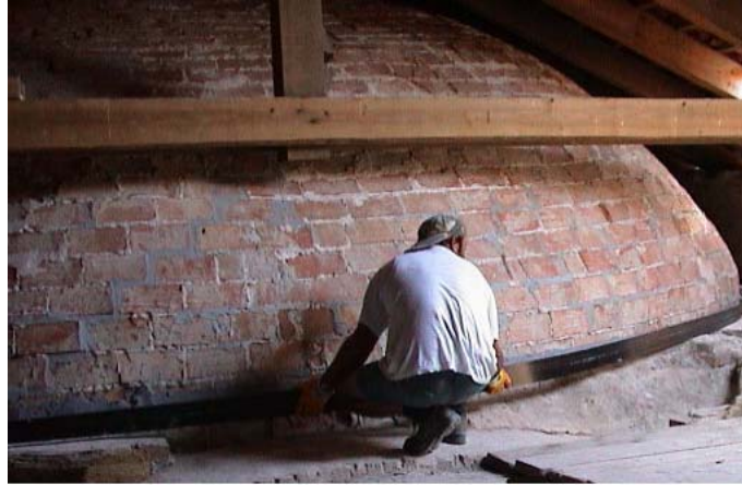
Figure 2.8. FRP strengthening of a masonry dome.
