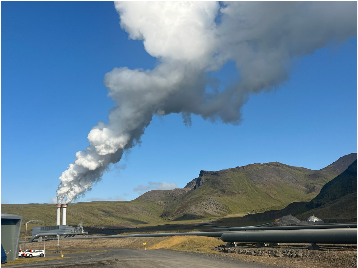
Hellisheiði Geothermal Power Plant in Iceland, 2023. / XAVIER BOLÓS
