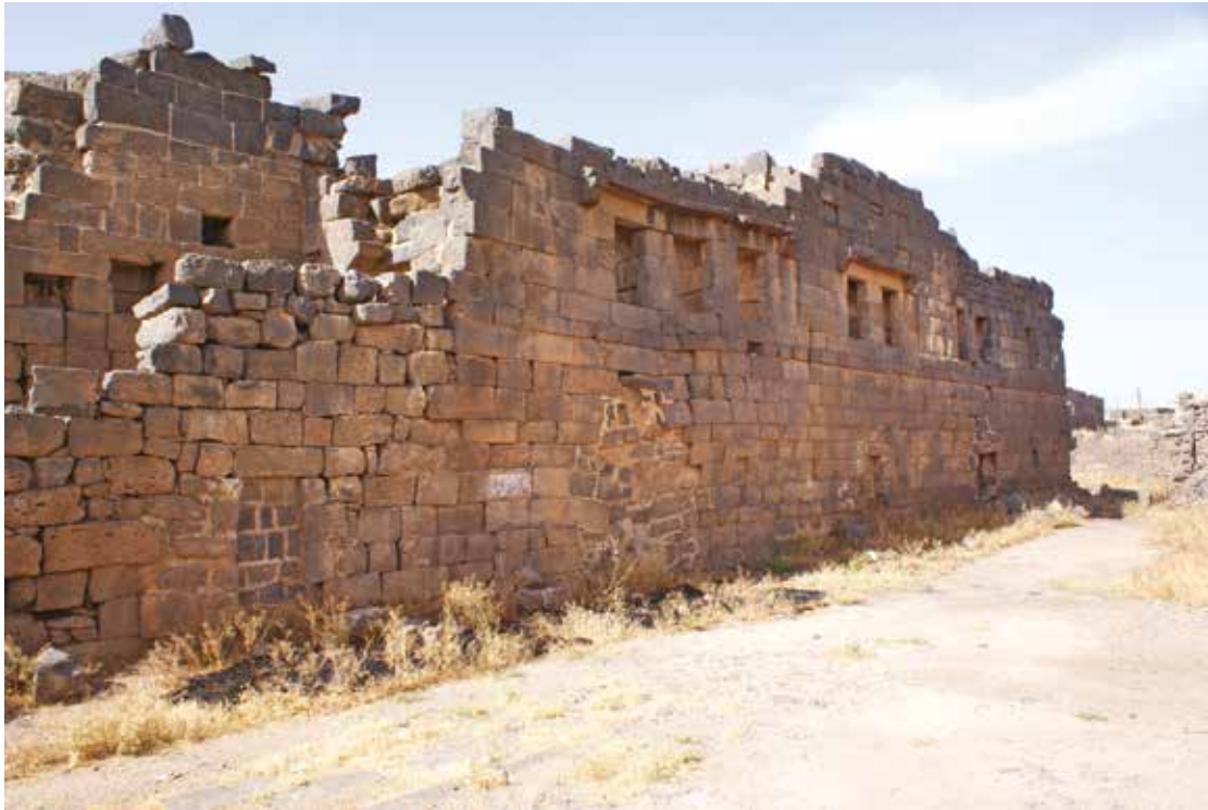
Fig. 2. Southern façade of the upper floors of the “Palace of Trajan” (The façade of the ground floor is still unearthed). © P. Piraud-Fournet 2016.
