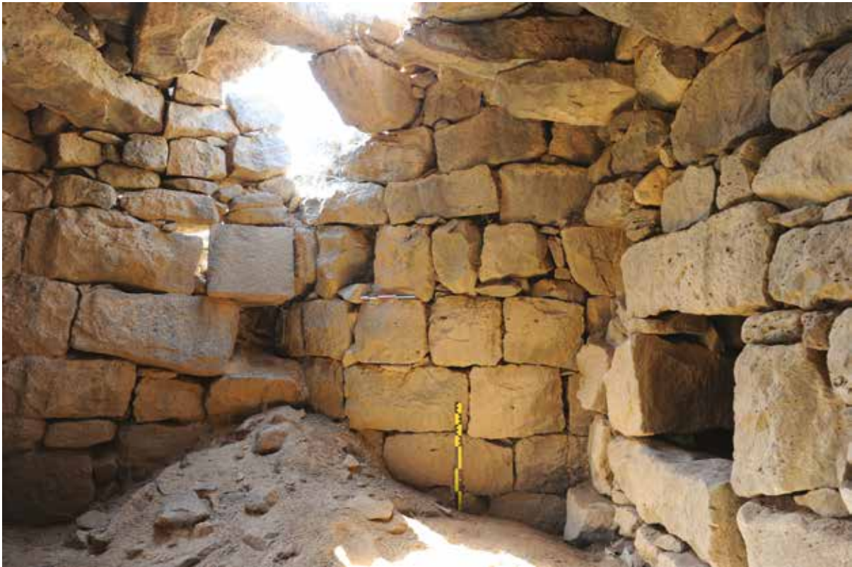
Fig. 11. Umm al-Surab. Two arches church. Partial view of the apse from the interior of a recent building (Photo by Piero Gilento 2018).
