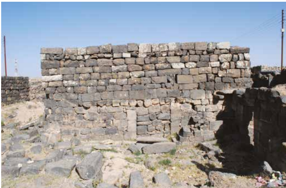
Fig. 15. Umm al-Qutayn. North-east church, façade (Photo by Piero Gilento 2017).
