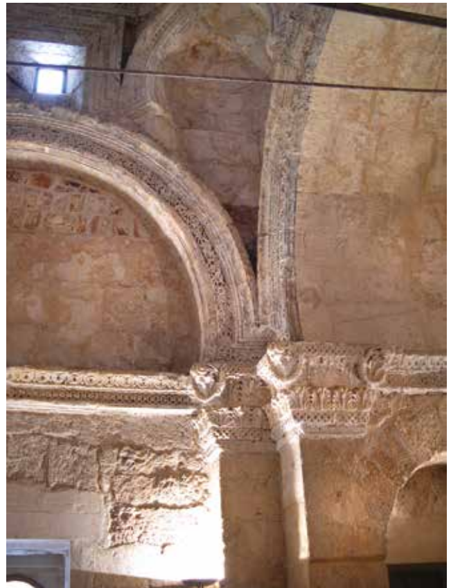
Fig. 19. Arches and capitals in the Church of Yoldath Aloho at Hāh.
