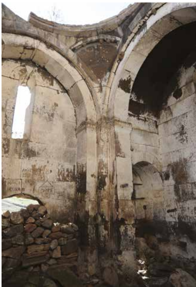
Fig. 11. Horomos Monastery, Surb Minas. Interior. Photo by A. Kazaryan, 2013.
