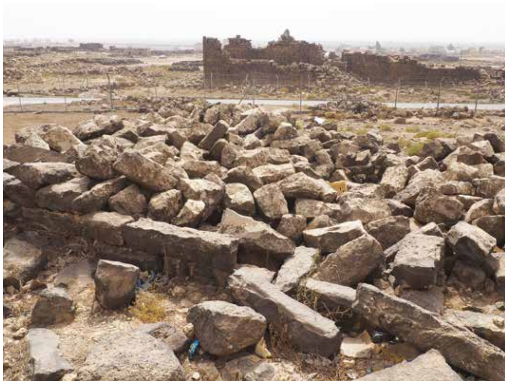
Fig. 10. In the foreground, Collapsed Annex Building of the Northern Church. © P. Piraud-Fournet 2018.
