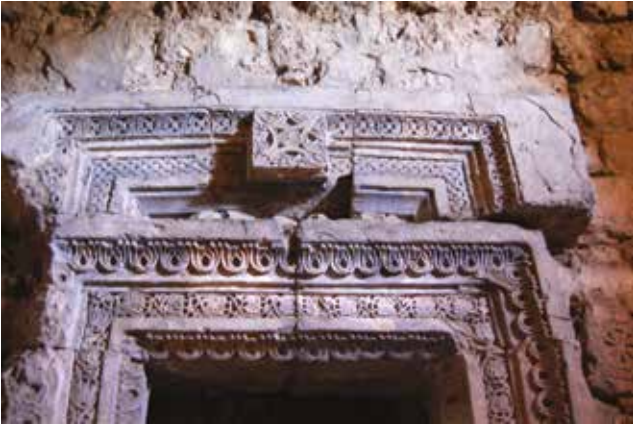
Fig. 27. Entrance to the apse in the Church of Mor Samuel at Hāh.
