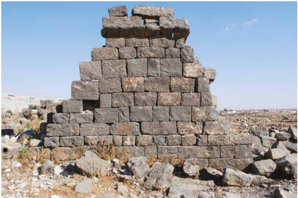
Fig. 6. Umm as-Surab. North church, façade (Photo by Piero Gilento).
