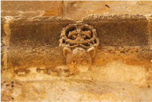
Fig. 8. Lion head on the cornice of the southern façade of the Church of Mor Ya'qub at Ṣalaḥ.
