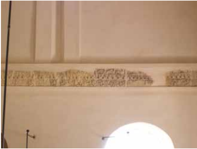
Fig. 4. Cornice under the vault in the Church of Mor Hananyo in Dayr al-Za'farān.
